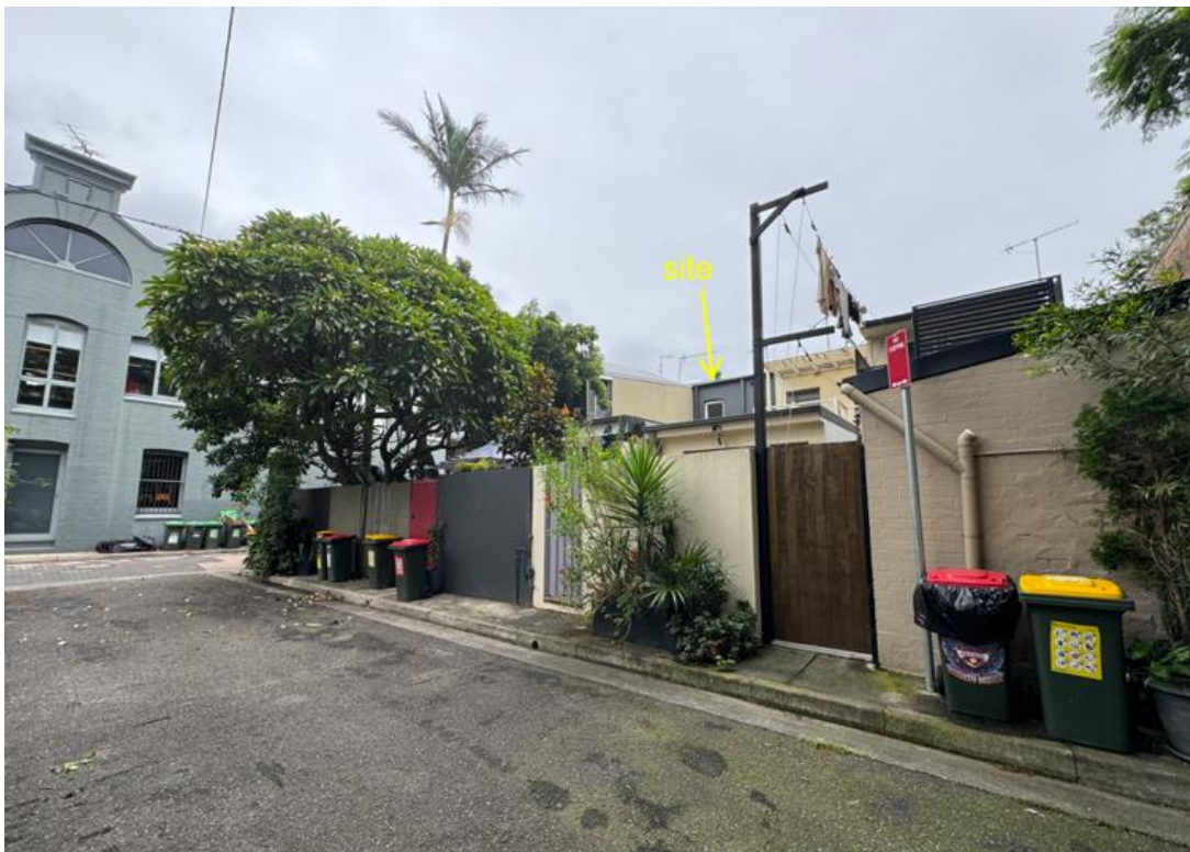
Figure 5: Site viewed from the Unnamed Lane
